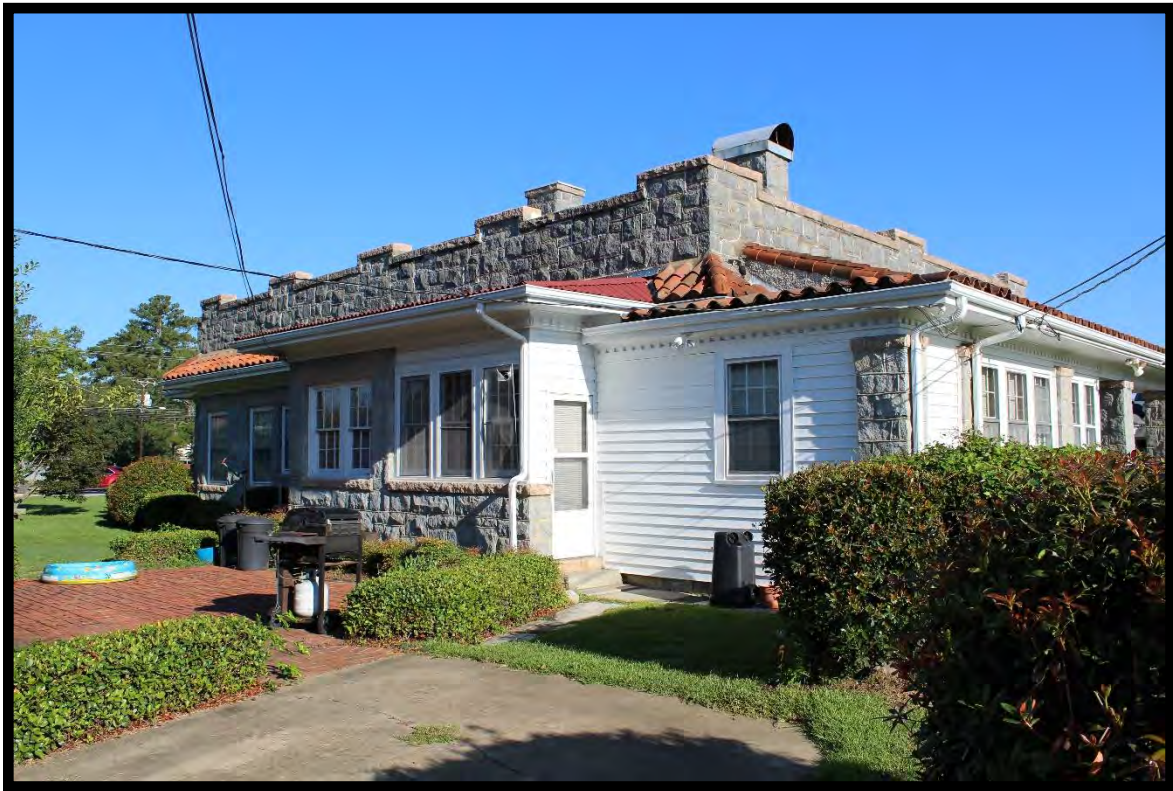
Figure 8: Cooper House, Looking Northwest (South Elevation).
