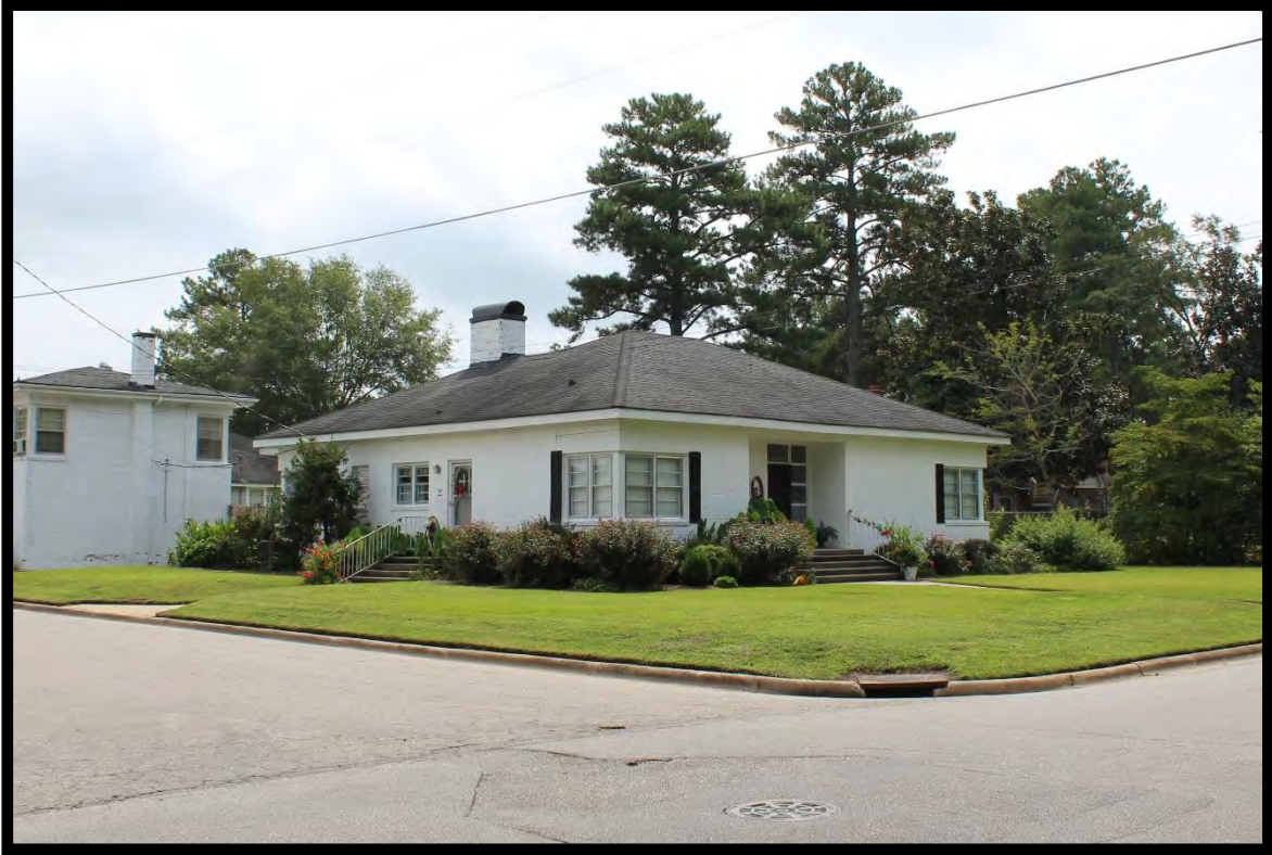
Figure 21: Wilson House, Looking Northwest (North and West Elevations).
