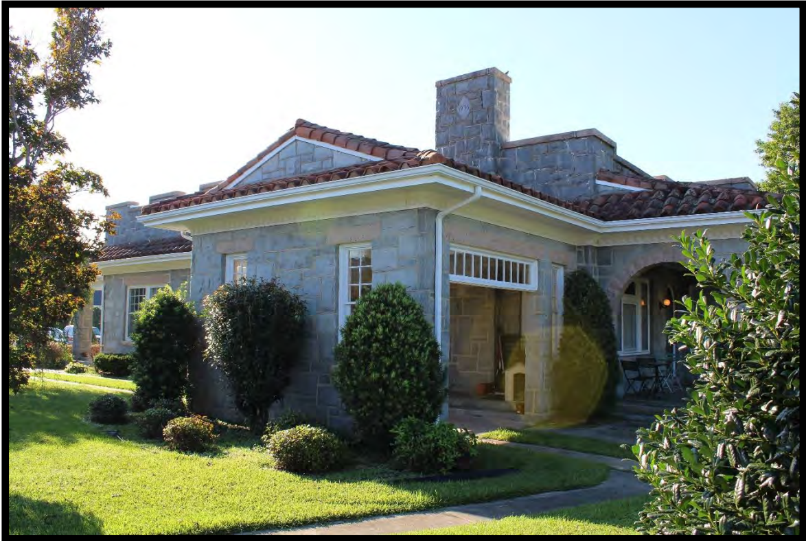
Figure 10: Cooper House, Looking Southeast (North Elevation). Note Datestone on Chimney.
