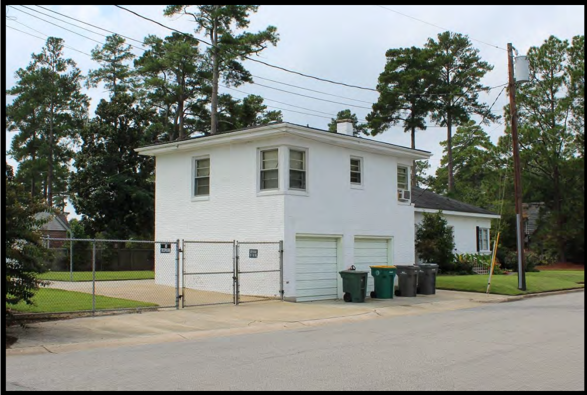
Figure 35: Wilson House, Garage/Apartment, Looking Southwest.
