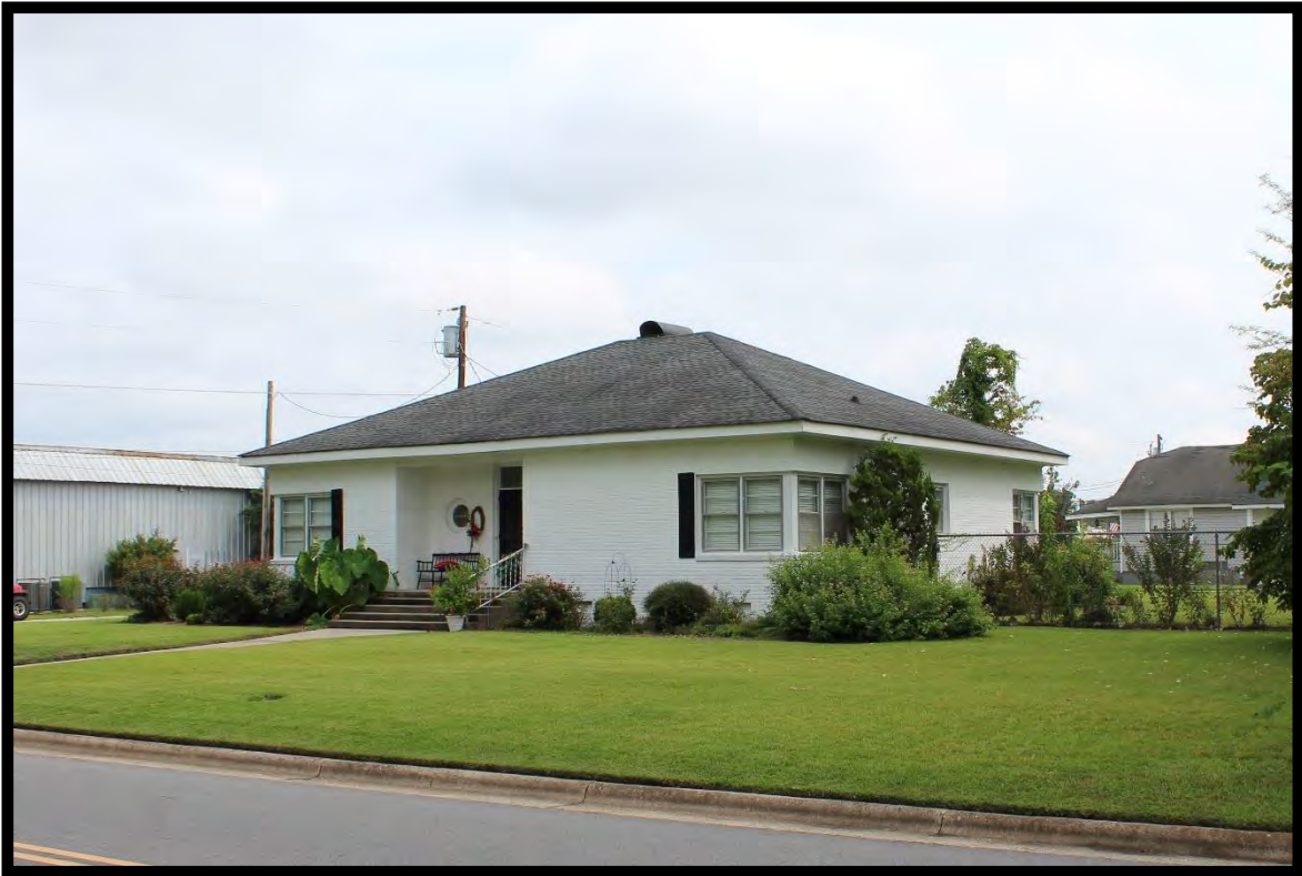
Figure 22: Wilson House, Looking Northeast (South and West Elevations).
