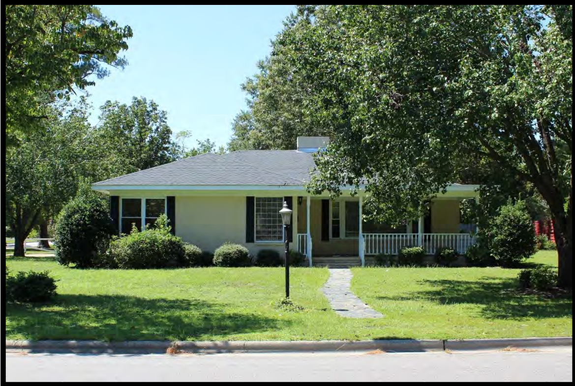
Figure 38: 2401 N. Rowland Avenue. Note corner windows, recessed entry and low slope, hipped roof.
