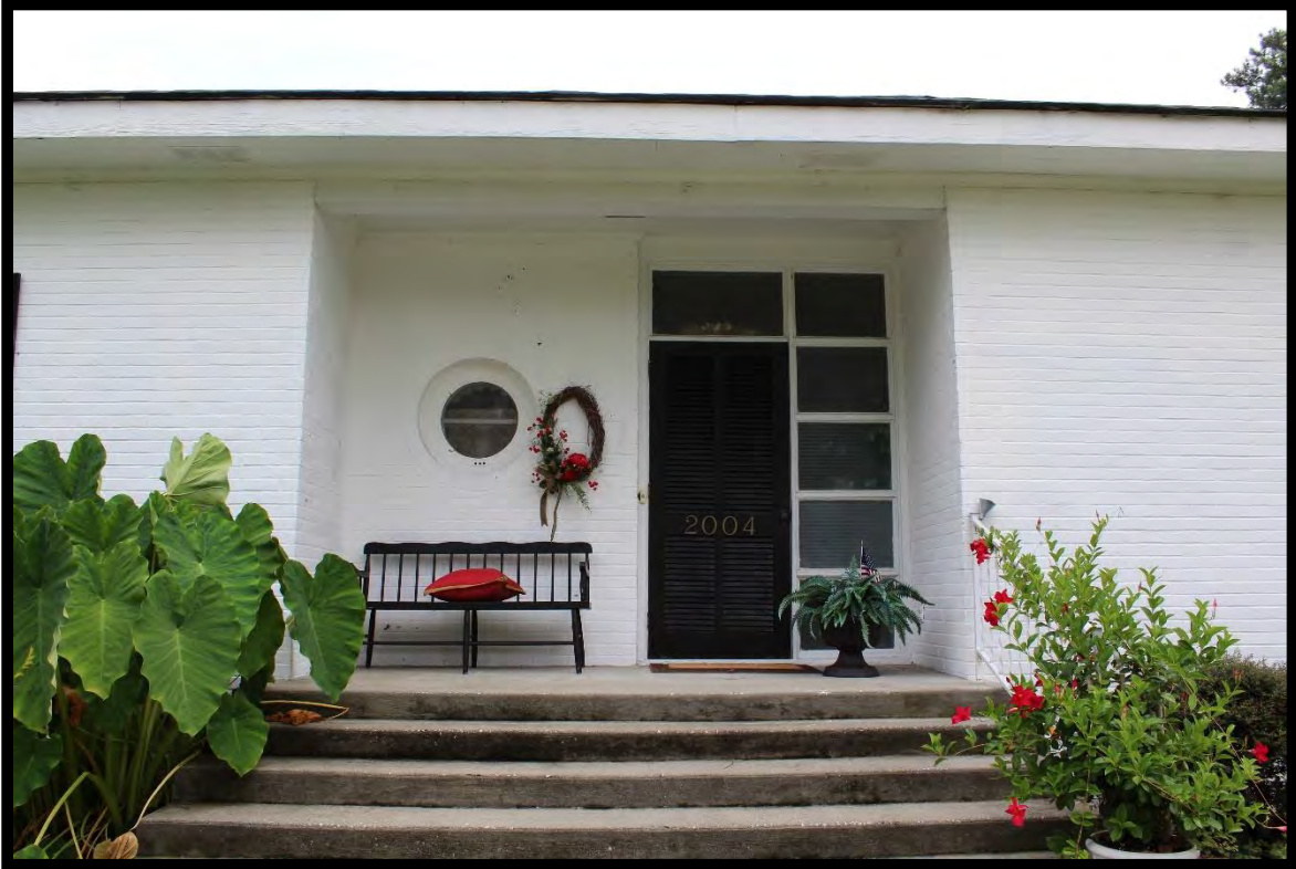
Figure 26: Wilson House, Detail of Recessed Porch, Looking East.
