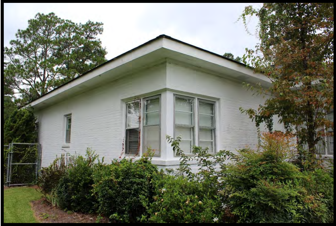
Figure 27: Wilson House, Detail of Corner Windows, Looking Northwest.
