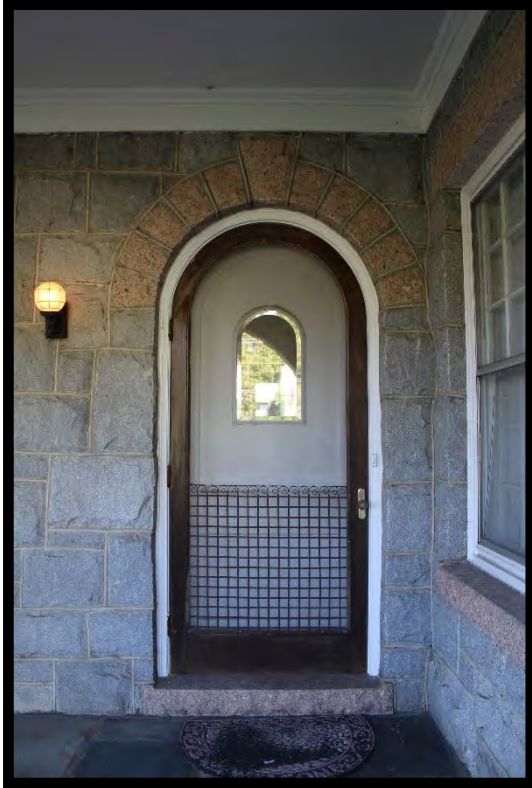
Figure 11: Cooper House, Front Entrance.
