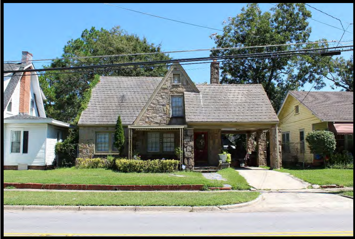
Figure 16: 1306 N. Pine Street, Looking East.
