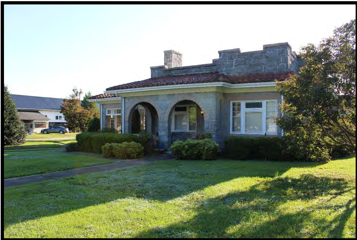
Figure 6: Cooper House, Looking Northeast (West Elevation).
